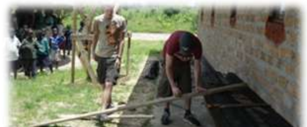
Tim surprised himself at his ability to make scaffolding!
